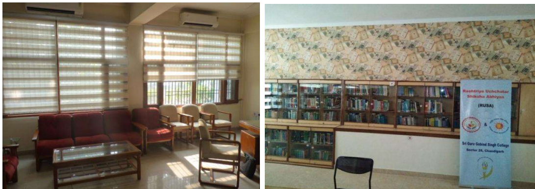
Installation of Blinds (Principal Office)/ Wallpaper In Library
