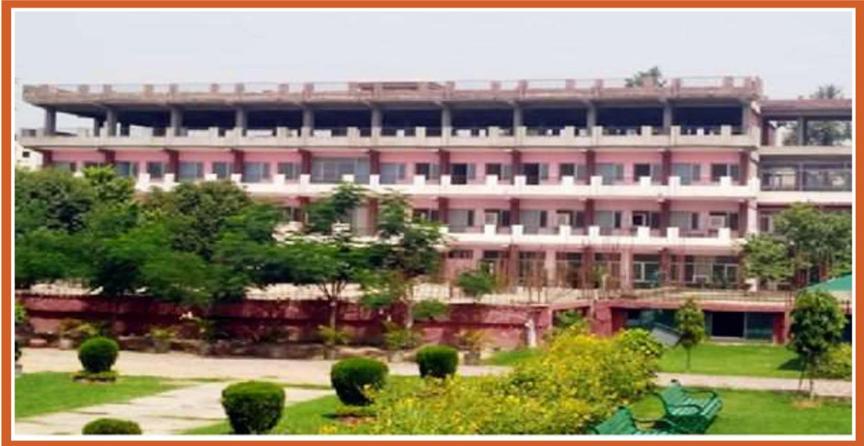
Strengthening of Hostel Infrastructure Resource Under RUSA Scheme at Dev Samaj College for Women, Sector-45, Chandigarh
