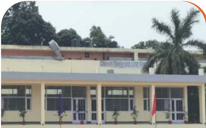
Construction of Classrooms under RUSA grant at Sri Guru Gobind Singh College, Sector-26, Chandigarh
